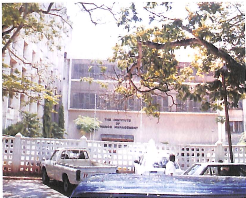
The Institute as seen from Samora Avenue, Dar es Salaam
